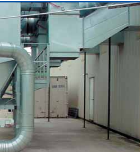
The Cabinet Door Shop's dust collection unit is totally enclosed so there is no sawdust accumulation, says Wheeler.
